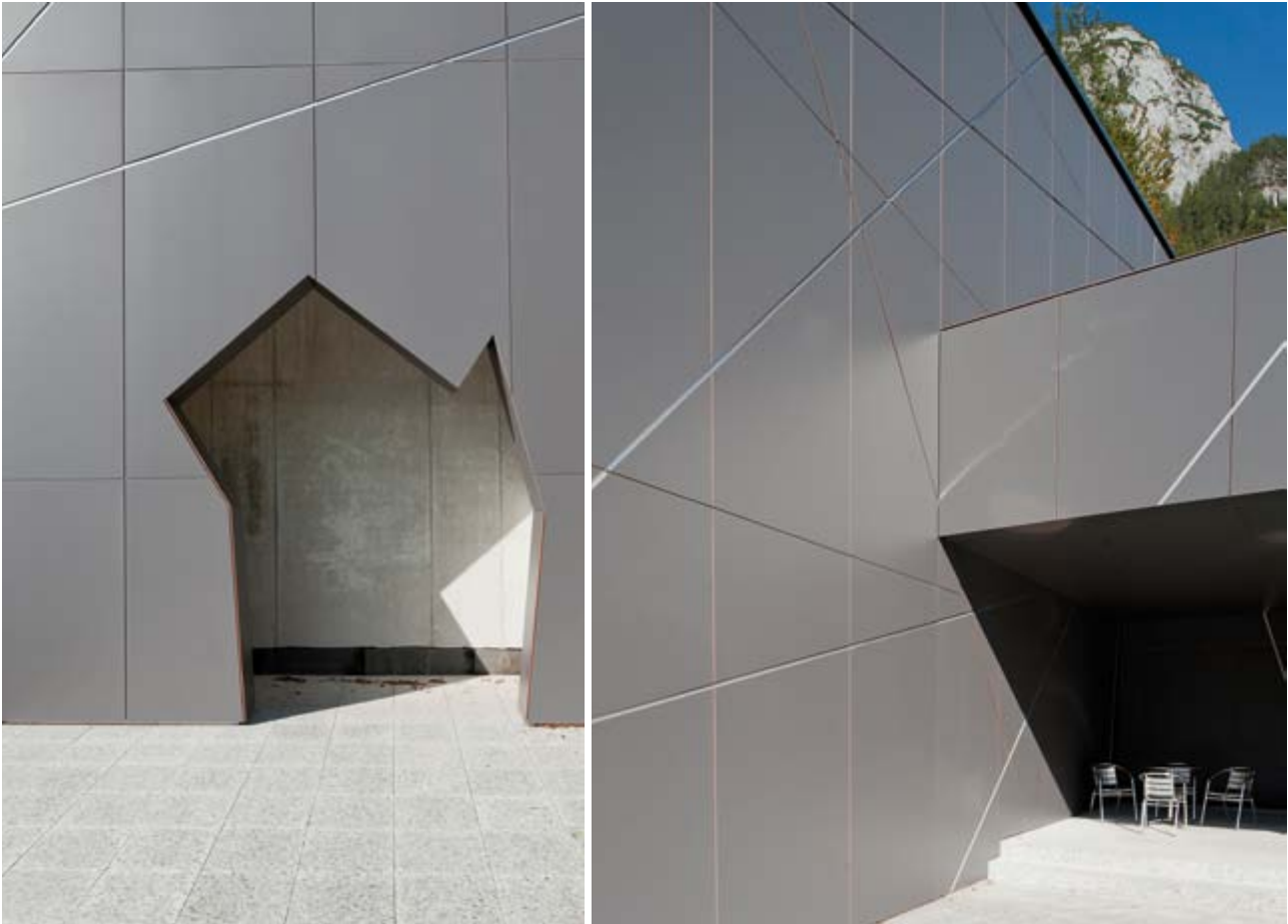
Project __Visitors' center Eisriesenwelt Werfen Country __Austria Design __Architect Werner Schmid Images __Angelo Kaunat Decor __0077 NT
